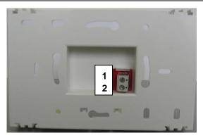
1 COA OpenTherm terminal A (interchangeable) 2 COB OpenTherm terminal B (interchangeable)
